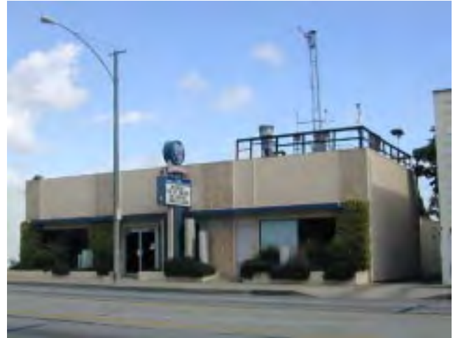
Exposed roof equipment is prohibited.
